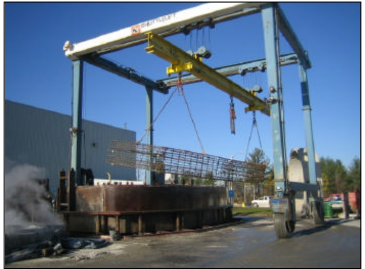
Mobile crane places cage into mold
