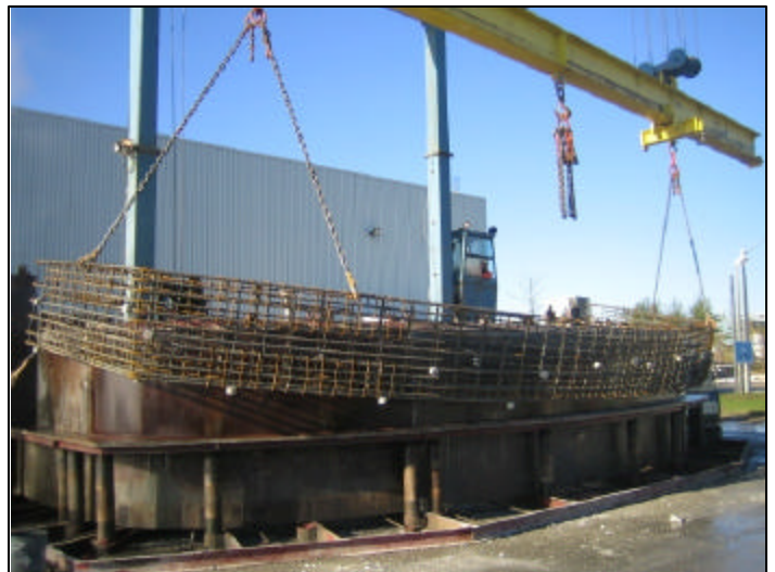
Placement of rebar cage in mold with a span of 10.98m and vertical rise of 3.96m.
