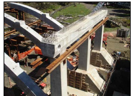
SSR used in bridge superstructure
