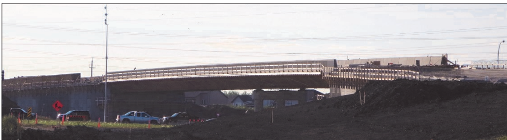
Two-lane overpass with two spans and a length of 104 metres.
