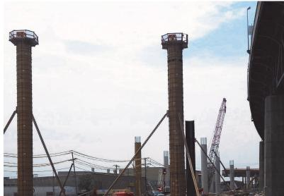
As of June 28, Brooklyn Rebar, LLC had taken delivery of approximately 60 tons for pier caps, 20 tons for an abutment wall and 1,000 tons of deck bars (#4,5,6) for the Brooklyn side of the structure.
