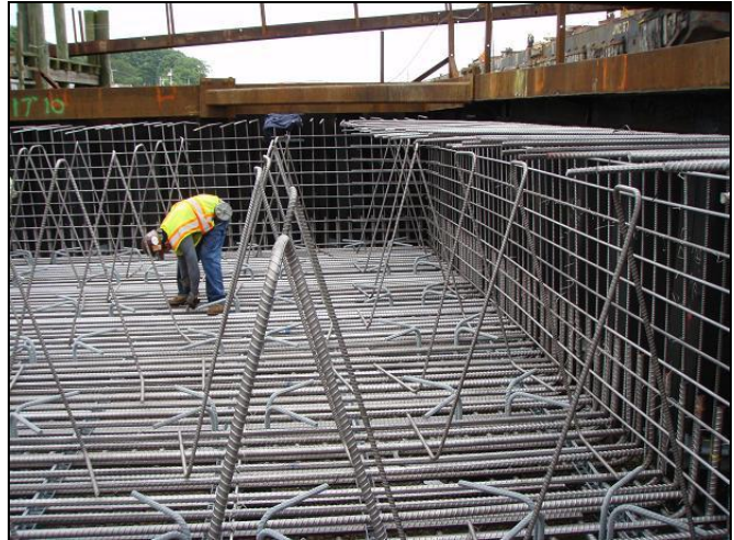
Rebar being assembled on site (Photo: Barker Steel LLC)
