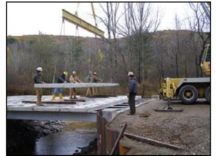
Galvanized girders support precast slabs on Allegany 20 bridge.
