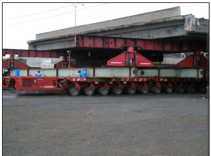
Old structure removed intact to make way for new bridge.
