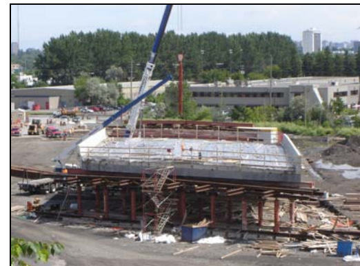
Bridge deck sections built separately in staging area.
