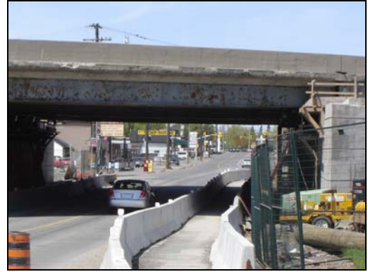
Old bridge deck being prepared for removal.
