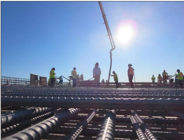
400,000 pounds of stainless steel type 2304 rebar used for the deck, barrier walls approach slabs and abutments.
